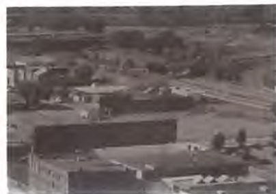
2016 aerial view looking west
