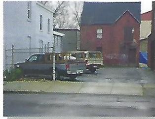
456 (was #106) Columbia Street Jensen/Kreber brick carriage house c.1907- 2019
