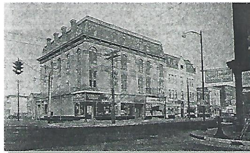
106 (456) Columbia St. c. 1956, now gone - light colored second building from the right and 110-112 Columbia St. the extant National Register eligible Witzberger Building - second from left - scheduled for demolition by MVHS. The four-story building on the left corner as St. George's Hall- now gone.
