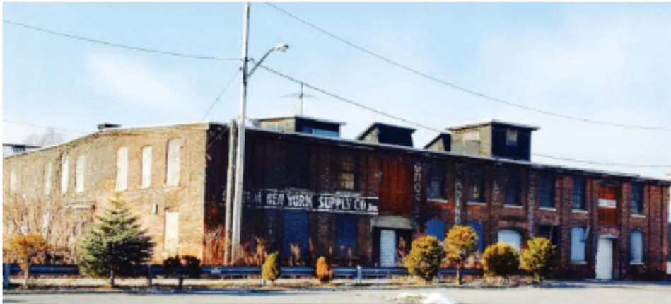
Citation Services, looking southwest from Oriskany Boulevard, 2018
